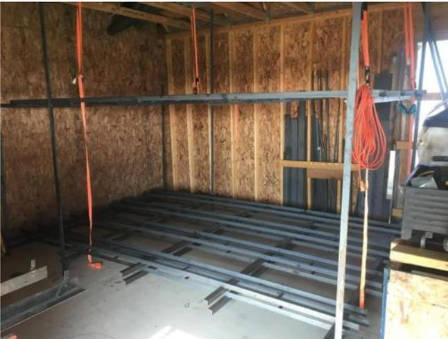
the ceiling joists), marked and drilled holes for the bolts and bolted them together, while checking for square and level. Then we proceeded to mark and drill the remaining bolt holes for the 6' verticals and bolt together. This was repeated for the middle level subassembly, and yet again for the bottom level subassembly, although clearances to get inside to drill the holes was a wee bit tight.
