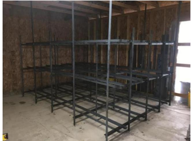
Checked for square and level again, then attached some 1" x 1/8" cross-brace strapping along the back.
