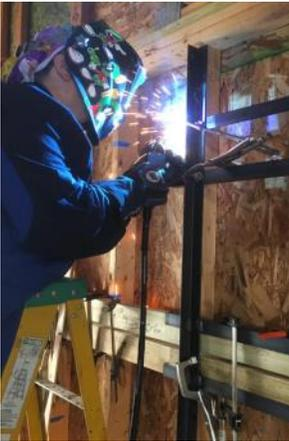
one from the back. This again allowed us to weld everything by standing up—not needing to crawling around on the floor. Each subassembly ended up with 144 welds.
