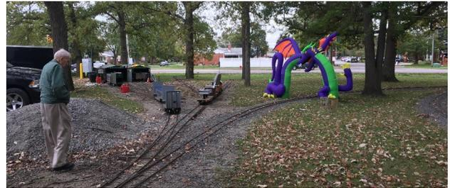
Their kidney-shaped 7.5" gauge track is approximately 3,000 feet in length uses profiled steel rail. It is on flat land and runs between the trees in the park. The mainline switches have frogs, while a few in their yard are stubs. All switches are manually controlled. The layout rests on approximately a 600x200 foot plot of land.
