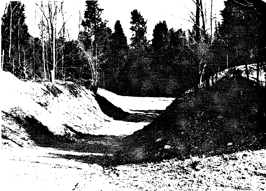
Once a wall of trees.....Looking Northeast from the end of the old parking lot, down the roadway that will be crossed by the covered bridge.
