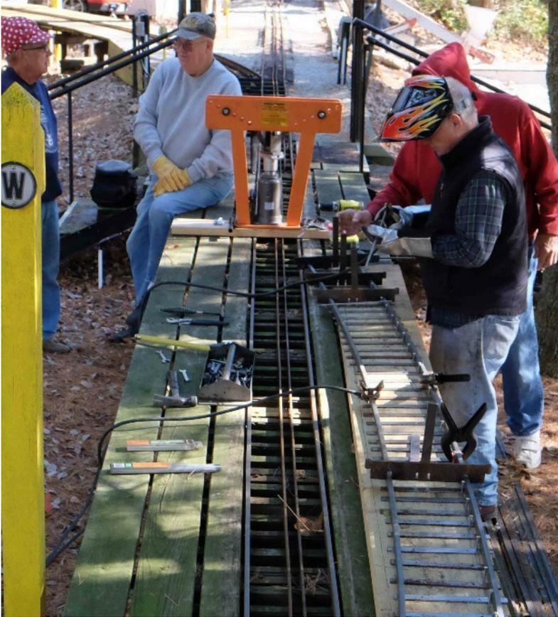
The second (inside) rail is then added using gauges to ensure 7½" spacing for 1½" scale rolling stock. Likewise, middle rails are added for ¾" and 1" scale.
