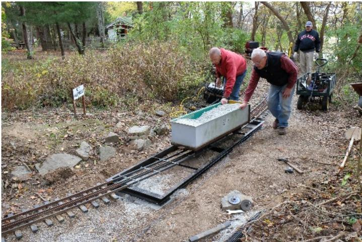
**Oct 22: The Test:** A section of the main line was cut out and in its place a “frame” upon which a “flexible track section” rests, both built by Carl Schwab, was installed in its place. Like all other turnouts on the property, the flex-track will serve as “switch points” when the turnout is completed.
